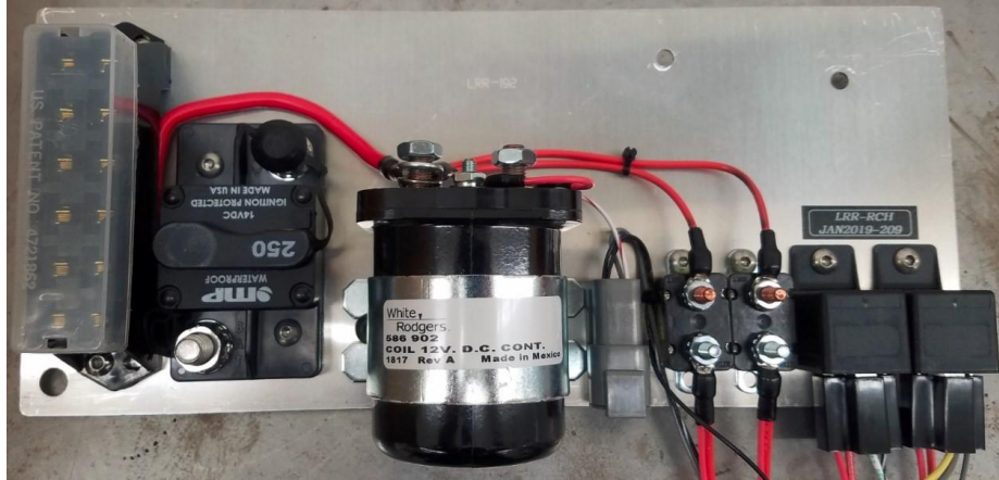
Figure 7: Power Distribution Panel (Trunk)
