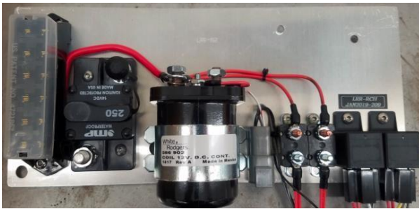
Rear Power Distribution Panel View 0000-08-D238
